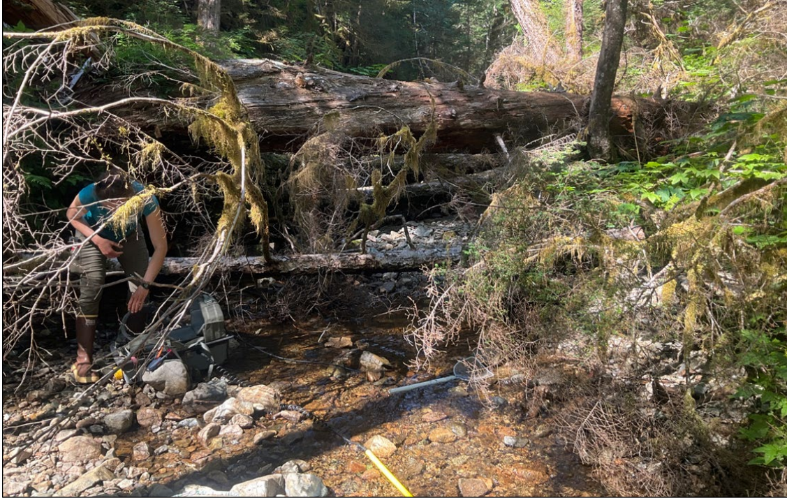
Figure 1. View of channel upstream at waypoint 488.
