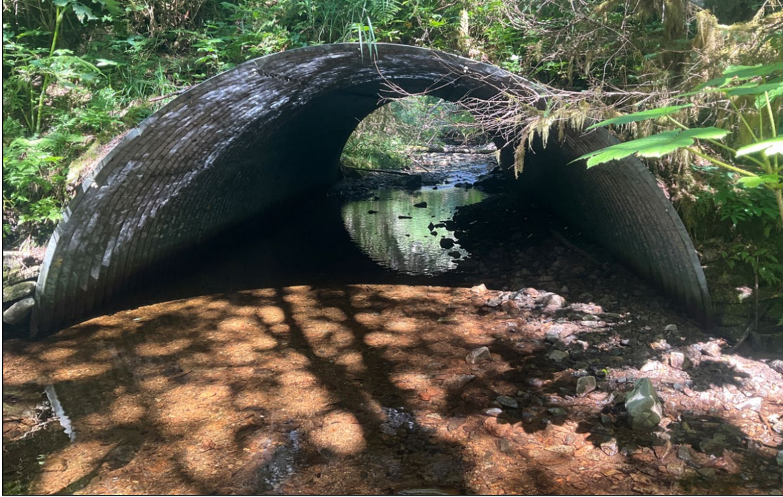
Figure 3. Culvert at waypoint 489.
